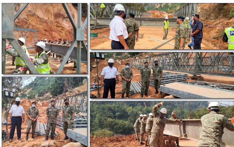
Malaysian Army builds Bailey bridge to SJSM, Hulu Terengganu
